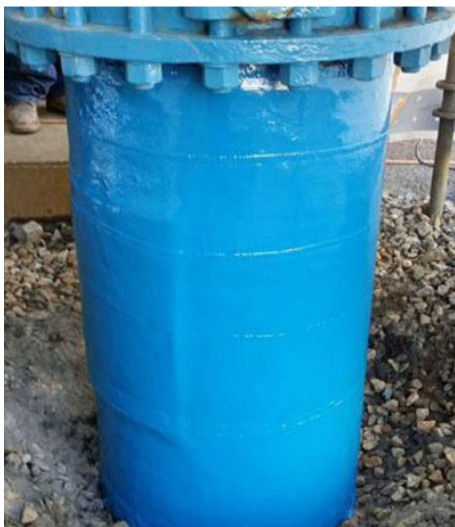
Vol 8 Issue 2 Coating Protection Applied to Chemical Containment Area
