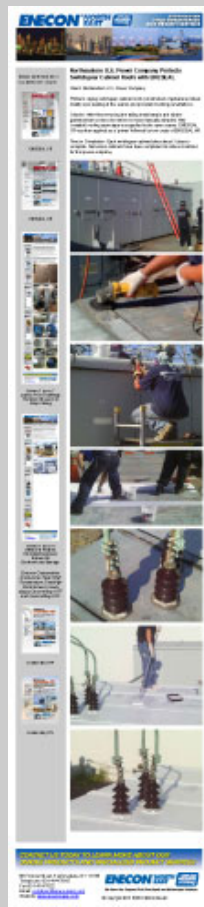
Volume 7 Issue 8 Sealed and Storm-Proofed Electrical Switchgear Cabinets
