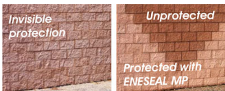
ENESEAL MP was initially applied in October, 2008.
