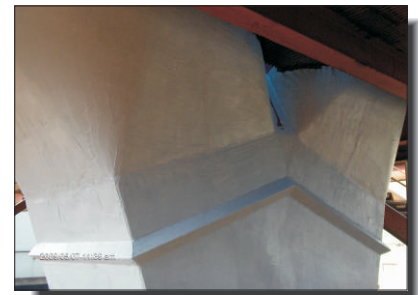
DurAlloy applied over entire extractor shell.
