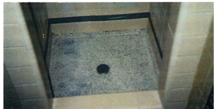
After all the surfaces to be protected are primed, the ENECRETE DuraQuartz application begins.
